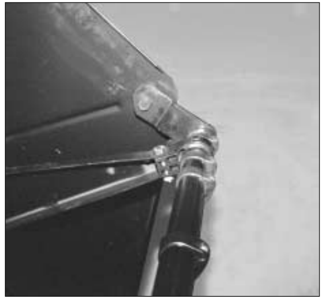
Illustration 17. Properly installed bat tube assembly.
